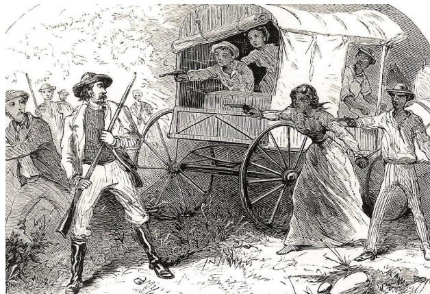
The fight at Hood's Mill
